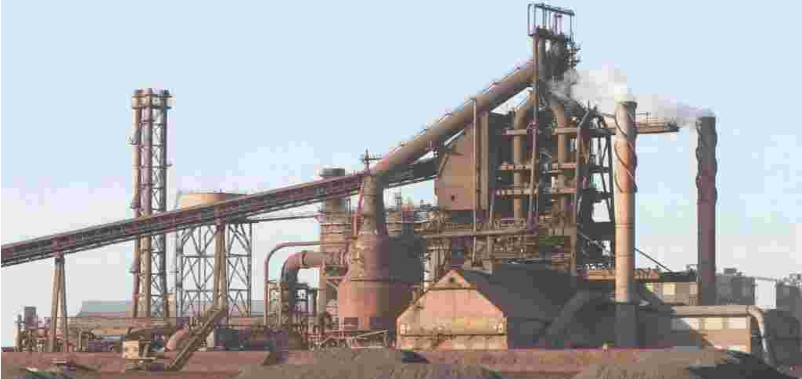
German Steel Mill .... Massive damage
